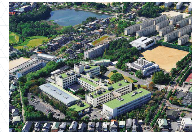
Panoramic view of the campus before renovations
